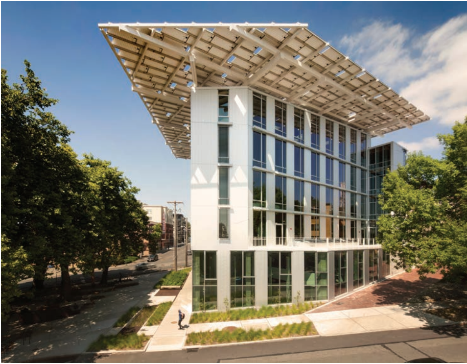
FIGURE 4-1. The Bullitt Center in Seattle is an example of a building designed to minimize its environmental impacts. Constructed of local materials selected for their low health and environmental impacts, the building has solar panels that generate as much energy as the building uses, employs geothermal heating and cooling, actively controls windows and shades to optimize natural lighting and circulation of fresh air, stores rainwater for nonpotable use, and has its own wetland to filter graywater.
