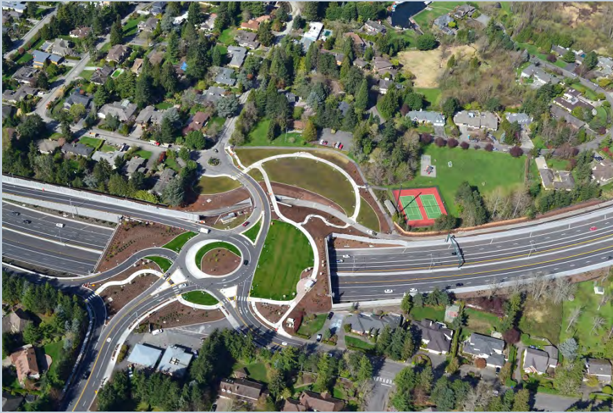
SR 520 Eastside Transit and HOV Project, Hunts Point, WA, photo courtesy of WSDOT.
